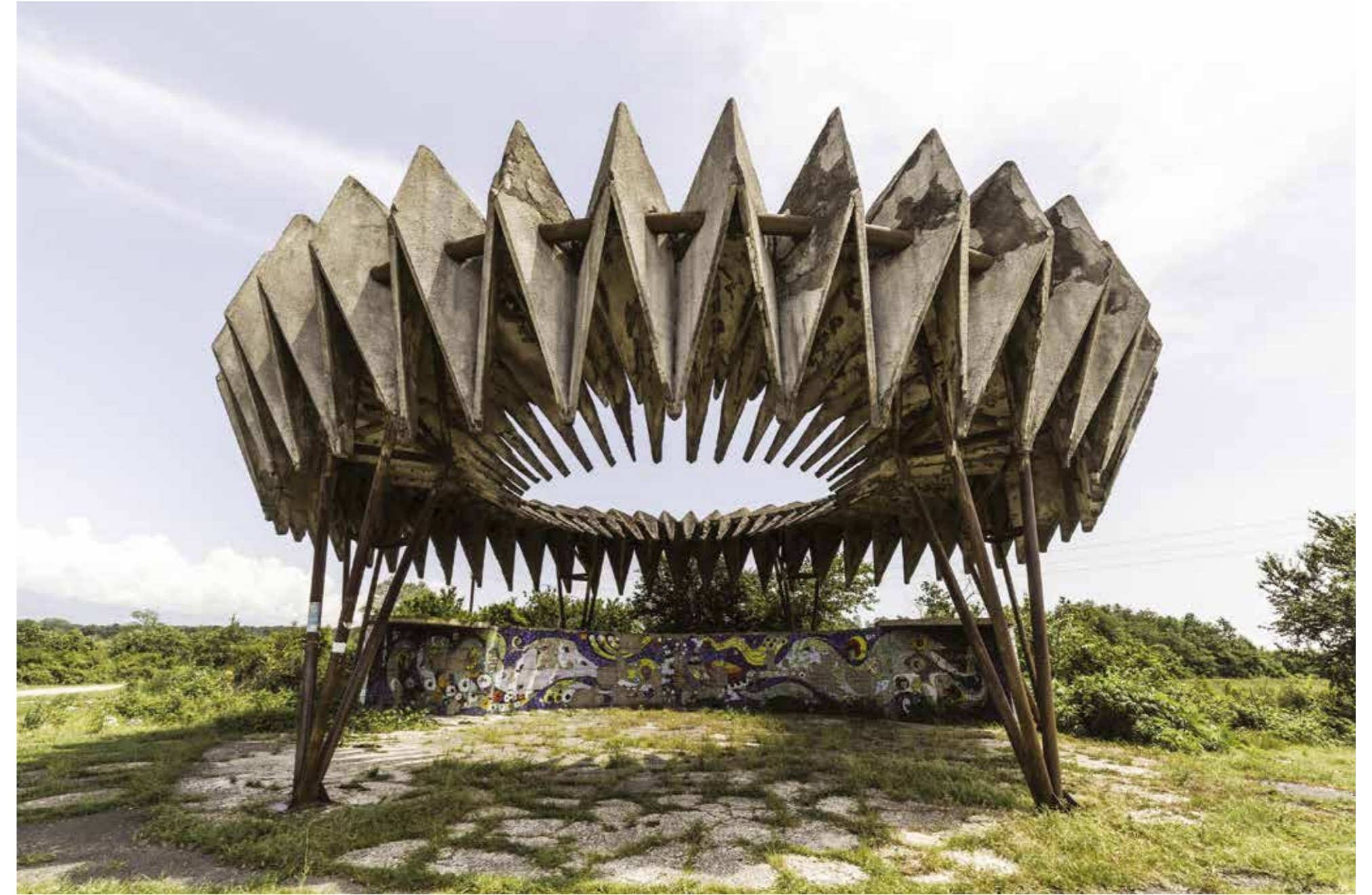
An eye-catching bus stop in the Brutalist style. Nowadays it is only the cows hanging out nearby that derive any sort of excitement from it.
